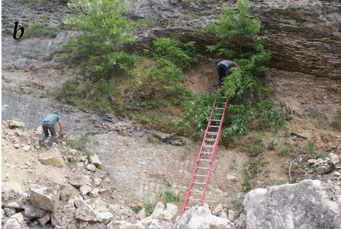
Figure 4. Work in 2019 to prepare the site for excavation
